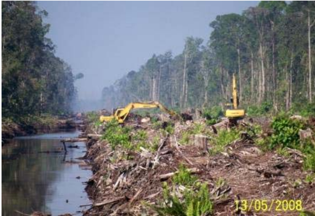
Image 1. New logging road construction by APP/SMG-associated companies in peat swamp forest of Senepis (N. 1 57 12 E, 101 13 15). It involves the clearing of a 50-meter swath of little-disturbed natural forest -- 25 meters width for the road and 12.5 meters width on both sides for drainage canals.
