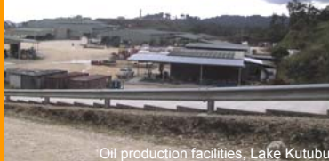
Oil production facilities, Lake Kutubu
